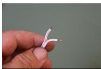
**8** Once a qualified electrician has established the intended wires run directly to an unpowered doorbell push button, remove a little of the insulation from the ends of the existing wires.
