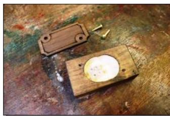
**6** Unscrew the junction box lid and remove the connector block.
