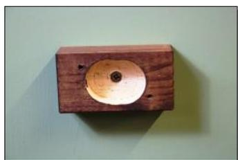
**7** As before, use the supplied screw and wall plug (if required) to fix the junction box to the wall, first checking there are no wires or pipes where the fixing will go. This time tighten the screw so the junction box is held in place.
